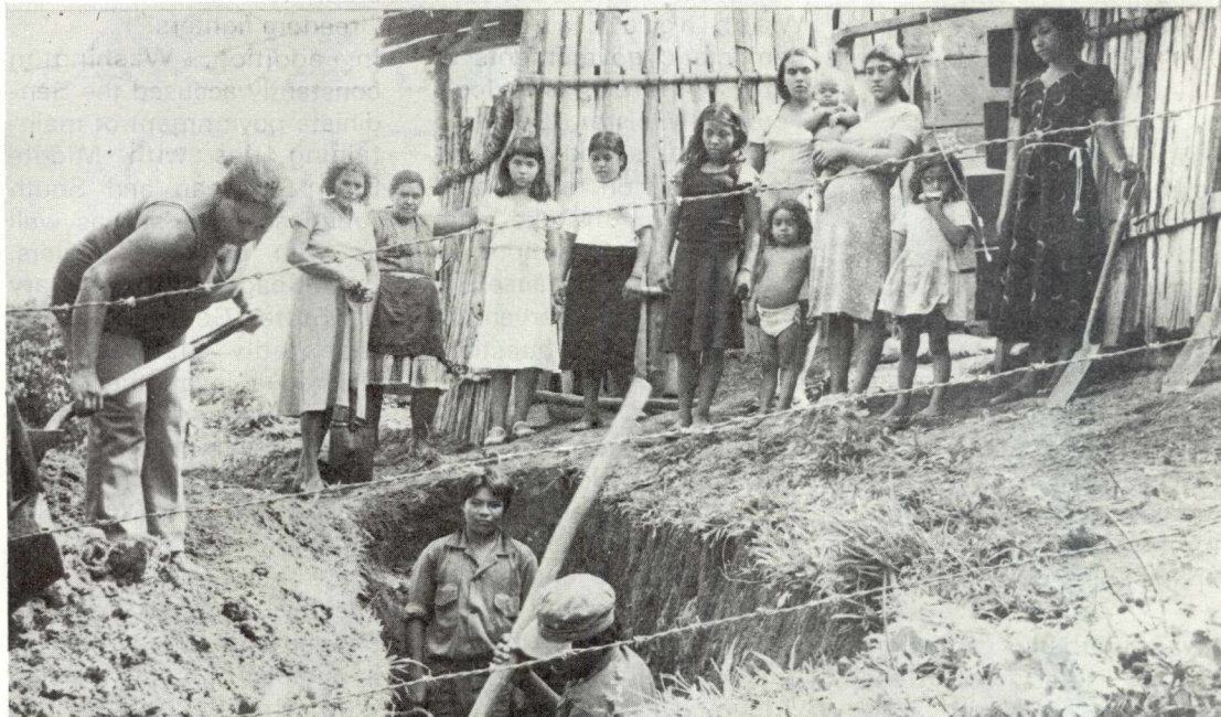
Civilian militias dig trenches to protect their homes in northern Nicaragua.
