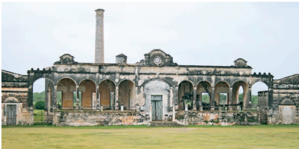
The engine room and the mechanical reaper room of Yaxcopoil, one of the biggest henequen haciendas in the early twentieth century.
