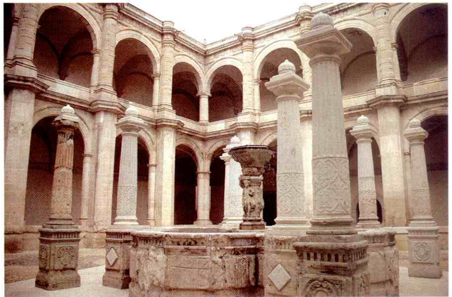
Restoring the building took more than 50 months of work.
