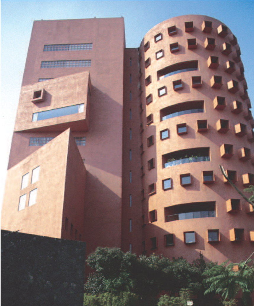
The National Center for the Arts' office tower has become a landmark in Mexico City.
