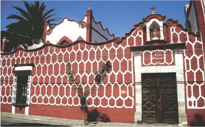
The Alvarado House today houses the Octavio Paz foundation.
