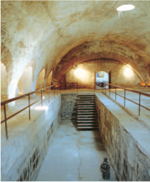
Santa Cruz Vista Alegre. Purging room.
