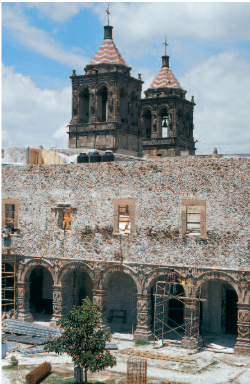
The Augustinian monastery complex was built during the seventeenth and eighteenth centuries, noted for the baroque in Mexico.
