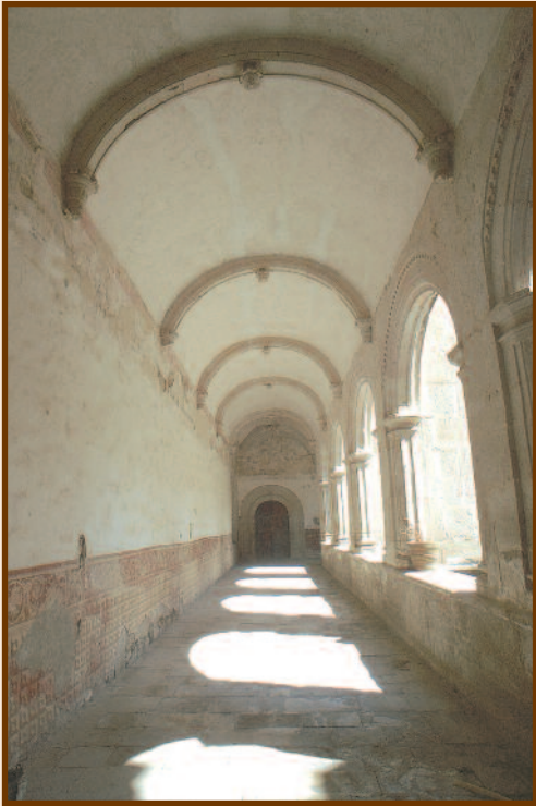
Cloister corridor, Saint Mary Magdalene Monastery, Cuitzeo.
