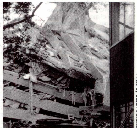
Some 300 apartments went down in the Nuevo León building, which became a symbol of the earthquake's victims.
