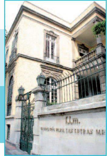
▲ The Foundation for Mexican Letters at 16 Liverpool Street.
