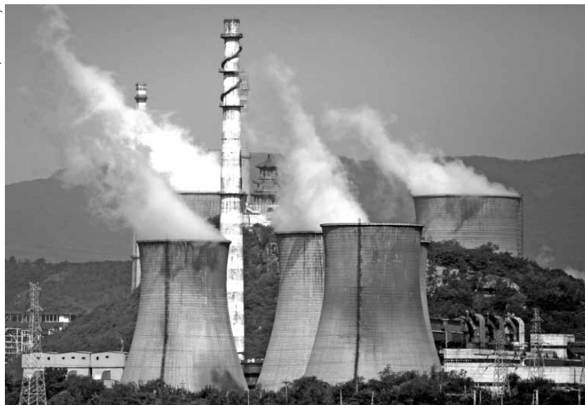
Environmental pollution from industrial processes also produces greenhouse gases (GHG) as well as damaging public health.
