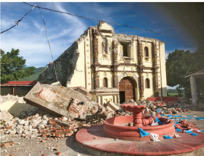
▲ Several churches in Jojutla, Morelos experienced the partial loss of structural elements like walls, vaults, and towers.
