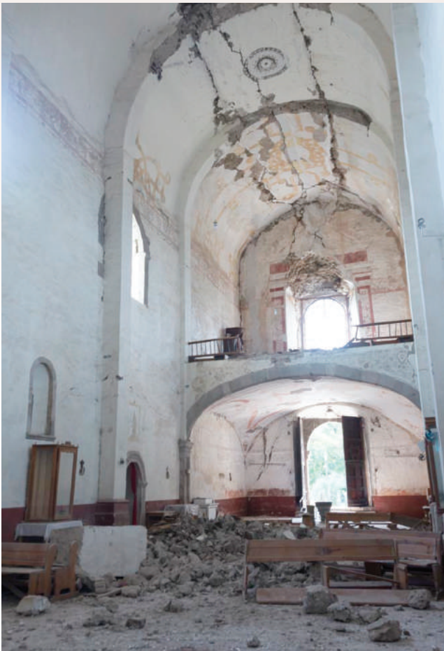
▲ Cracks and debris in the vault of the San Juan Bautista Church in Tlayacapan.
