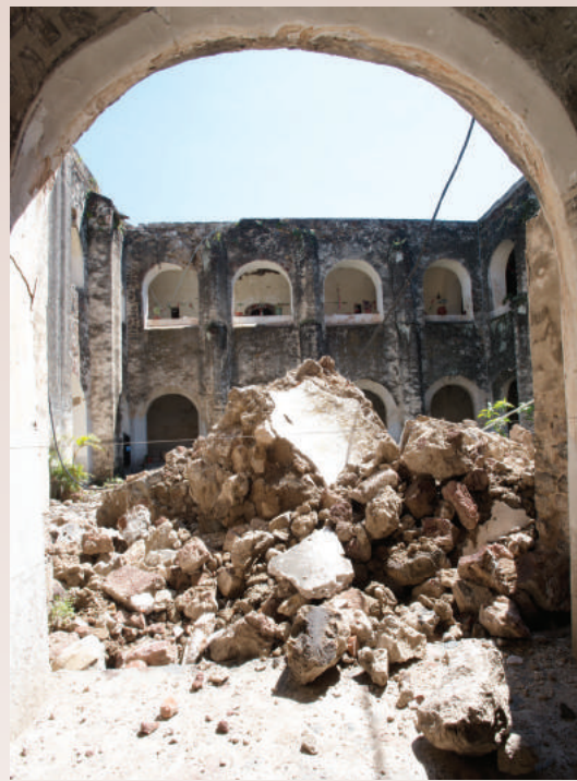
▲ Debris from the collapse of the west gallery of the upper cloister in Tototlan.
