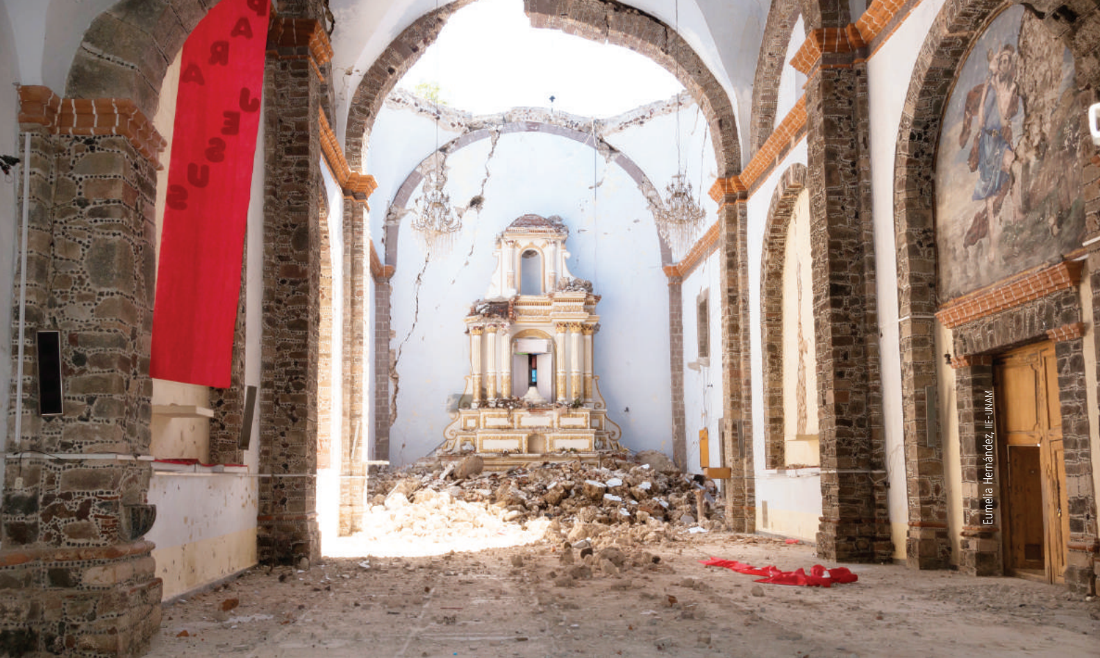
▲ Collapse of the dome over the high altar in the San Guillermo Totolapan Church.
