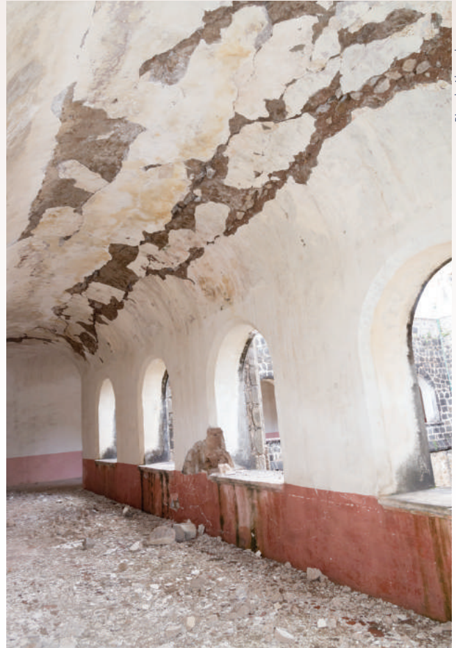
▲ Plaster detached from the mural painting on the vault of the former Tetela del Volcán Monastery.
