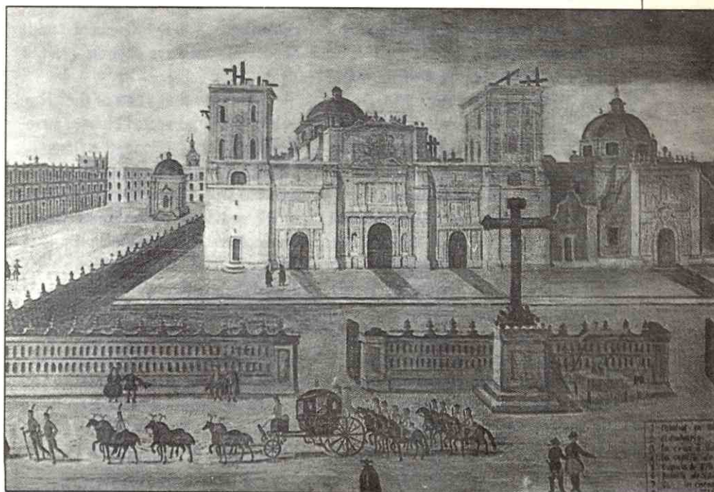
"The Cathedral Under Construction, 1764," anonymous work in the Franz Mayer collection.
