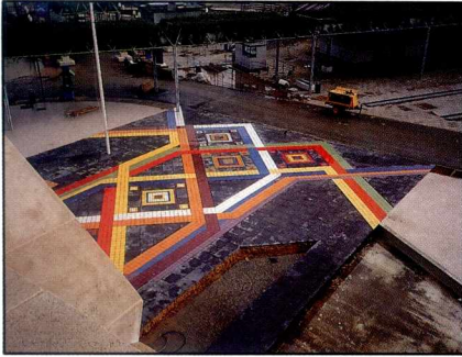
The Mexican Pavilion under construction.
