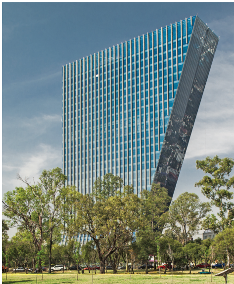
Teodoro González de León, Torre Virreyes (Viceroys Tower), Mexico City, 2010-2015. ▼
